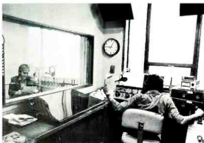
Bill Moos (top), operations director, at the studio A console. Note convenience of wall-mounted monitor pod containing remote control and monitors. Studios were designed with wheelchair access in mind.
